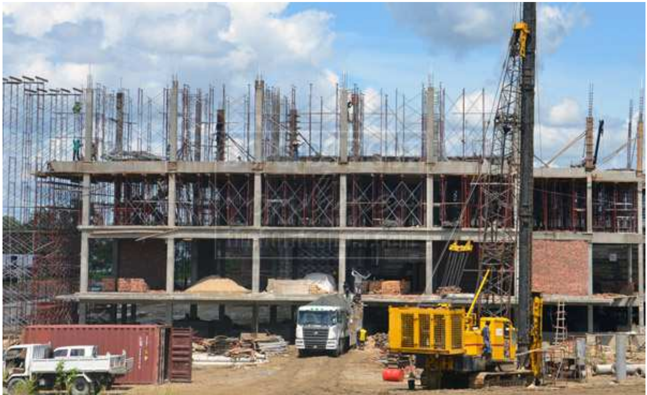
AHEAD OF SCHEDULE: One of UCTS buildings under construction.
